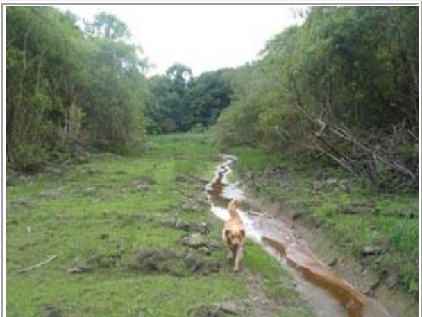
Drainage works on the upper lake
