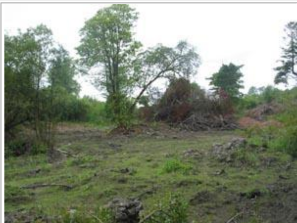
Drainage works on the lower lake
