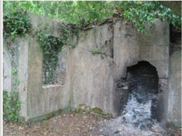
The old "Gazebo" or summer house which overlooks the lower lake. Picnics were held here and apparently it was also used for shooting Ducks from.
