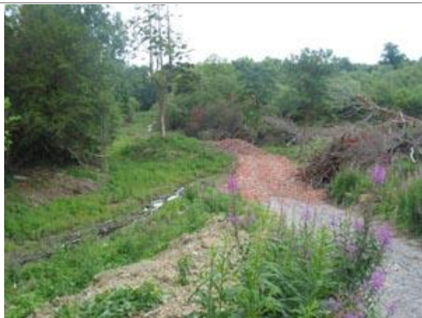
Drainage works on the lower lake
